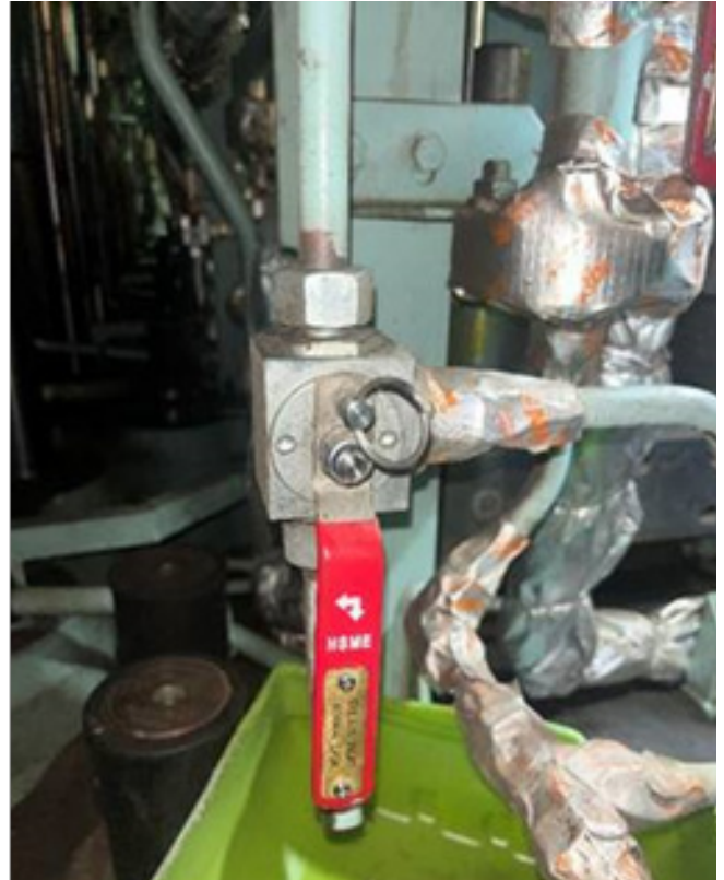
Fig. 3: Three-way valves without end-stops in an incorrect closed position, the necessary connection to the venting line has not been established
