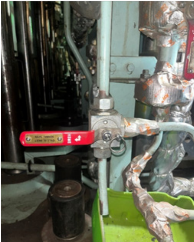
Fig. 3: Three-way valves without end-stops in an incorrect closed position, the necessary connection to the venting line has not been established
